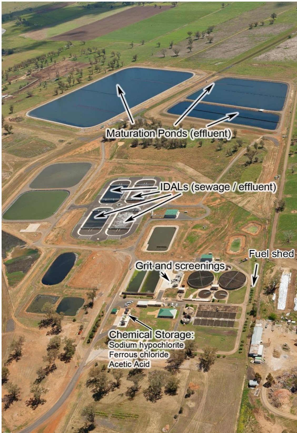
Westdale Waste Water Treatment Plant aerial view
